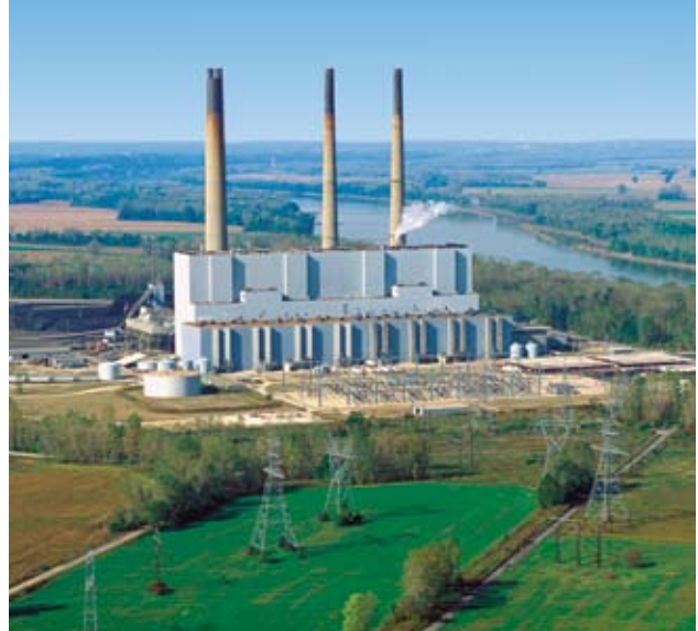
In terms of reducing nitrogen oxide emissions, AmerenUE's Labadie Plant units have often ranked among the top units in the nation among those that do not have selective catalytic or noncatalytic reduction systems.
